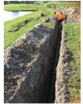
Temporary splitting of pump house output line to handle 2 systems
