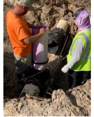
Temporary splitting of pump house output line to handle 2 systems
